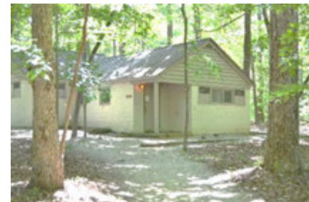
Demolish Existing Shower house
