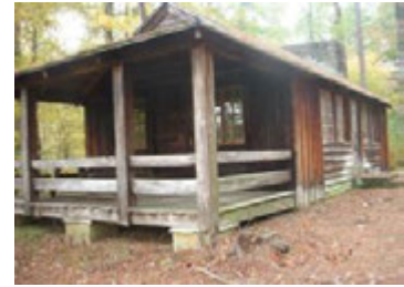
Camp Sycamore Lodge renovated for overnight use
