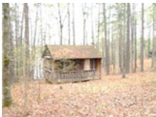
Condition of Structures - 2011
