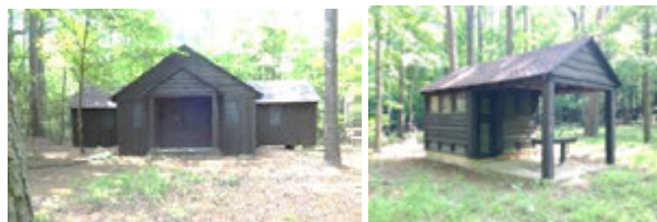
Structures after renovations
