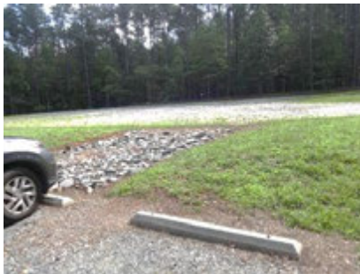
Existing Parking Lot expansion
