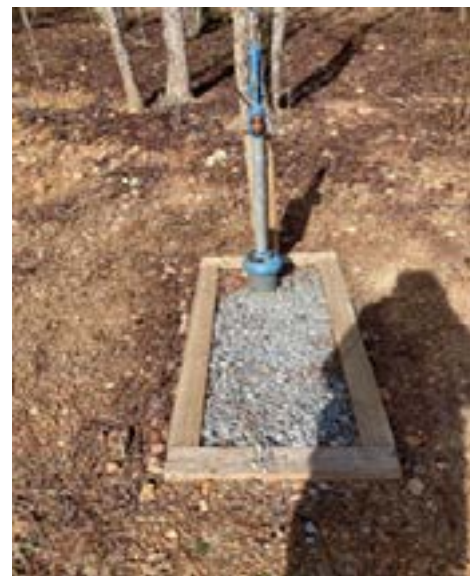
Proposed water spigot on impact pad
