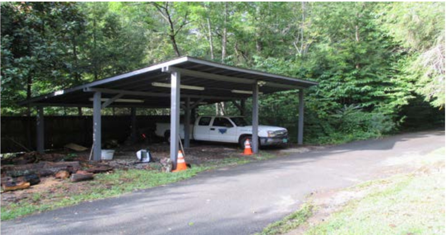
A proposed equipment storage building will provide additional storage area for supplies and equipment for the natural resources staff similar to the structure at Jacob Fork access at South Mountains State Park. The structure will have an open back and one bay enclosed.
