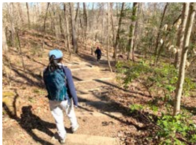
Wooden platform steps have been damaged by use and age.
