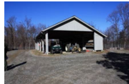
Existing Maintenance Storage Building
