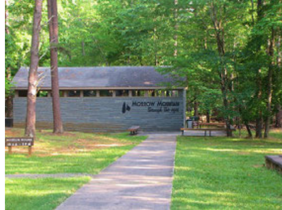
Museum located near the office, was constructed out of argillite stone mined in the park
