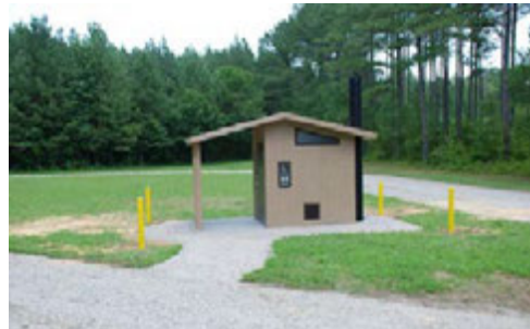
Vault Toilet in Equestrian area
