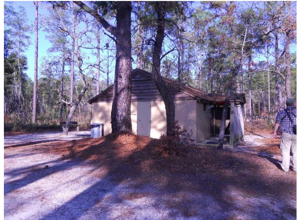
Existing Showerhouse does not meet clearance and will be demolished
