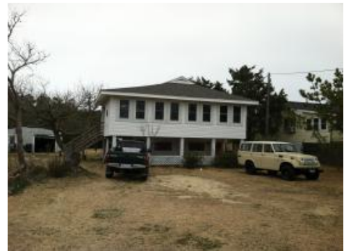
Park Residence built in 1970 that will be demolished
