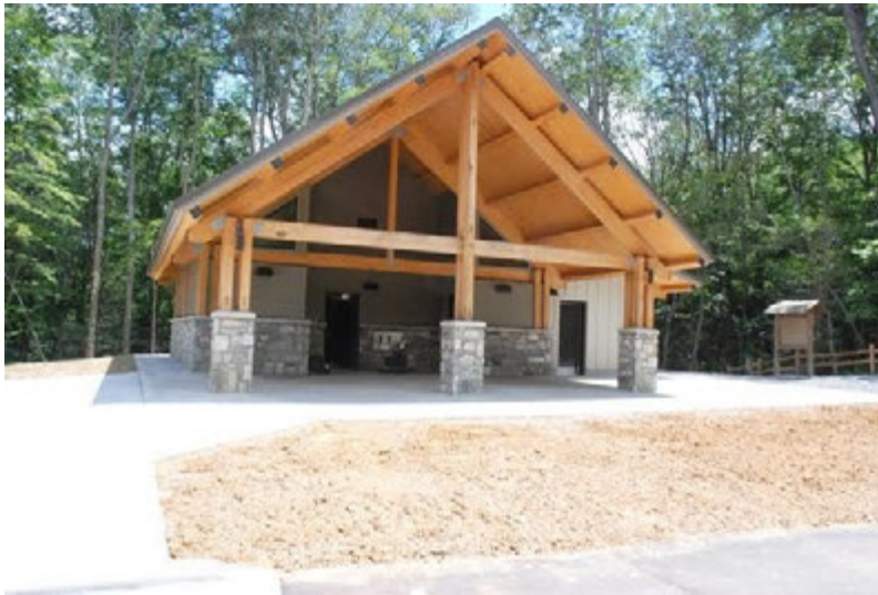
Restroom and Profile trailhead provides a centralized area for public and staff access. A contact station will be designed and constructed
