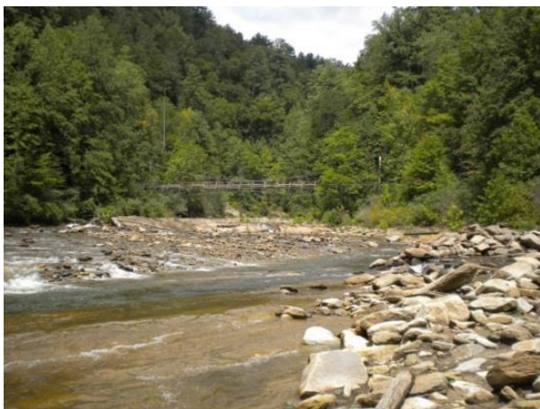
Foothills Bridge at Toxaway River
