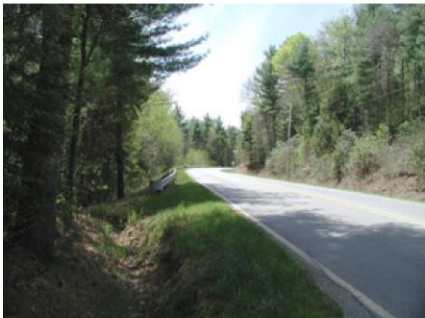
View south on NC 281 at new main entrance location
