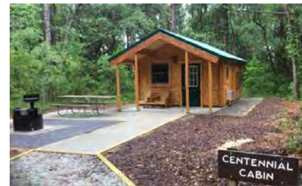
Standard Camper Cabin installed at Carolina Beach State Park
