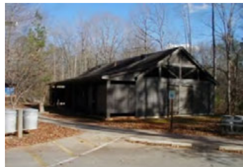
Holly Point Showerhouse Side View – Constructed in 1994. 1,152 sq. ft, wood frame, slab on grade
