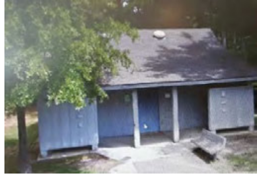
Existing Toilet Building.
