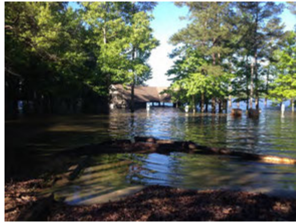
Sandling Beach Shelter No. 4 – 8 feet above Flood Stage
