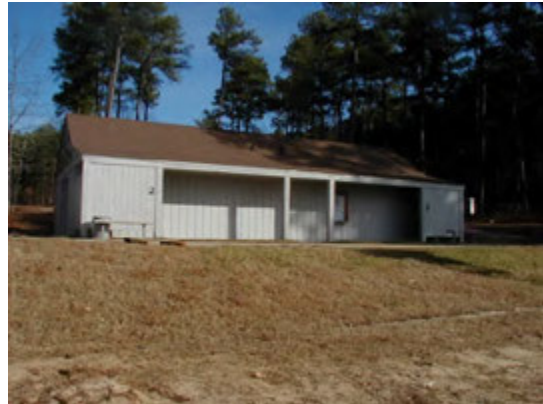
Rolling View Swim Beach Bath house Bldg# 040719, 1,131 sq. ft. wood frame, single story, slab on grade. Good condition.
