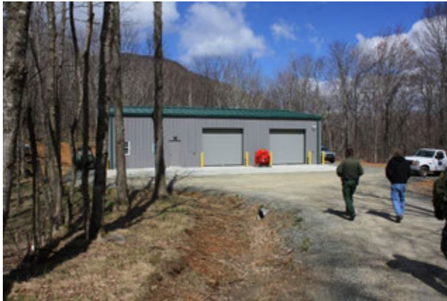
Maintenance Shop- Exterior
