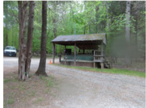
Existing Fueling Station
