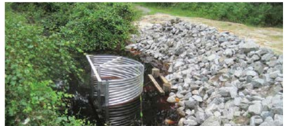
Water Control Structure
