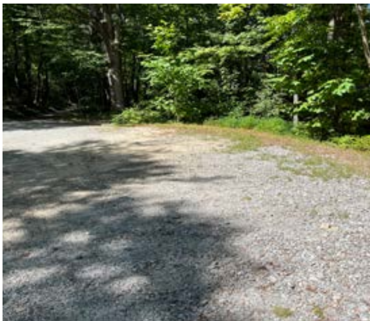
The existing trail head will be expanded to accommodate additional parking spaces
