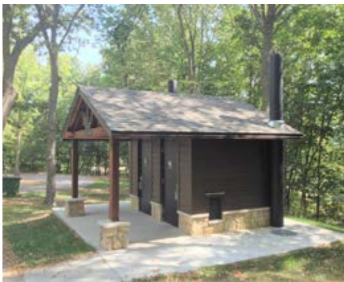
Prefabricated vault toilet will provide park amenities
