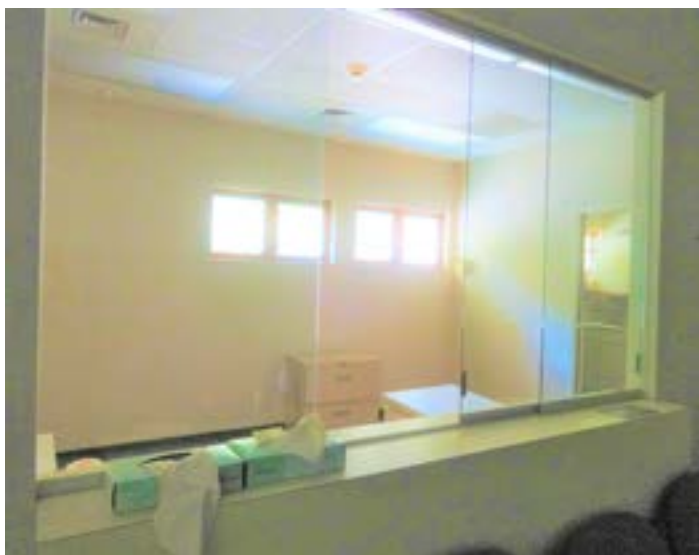
Former check in/receptionist area will be converted to an office administration space or workroom
