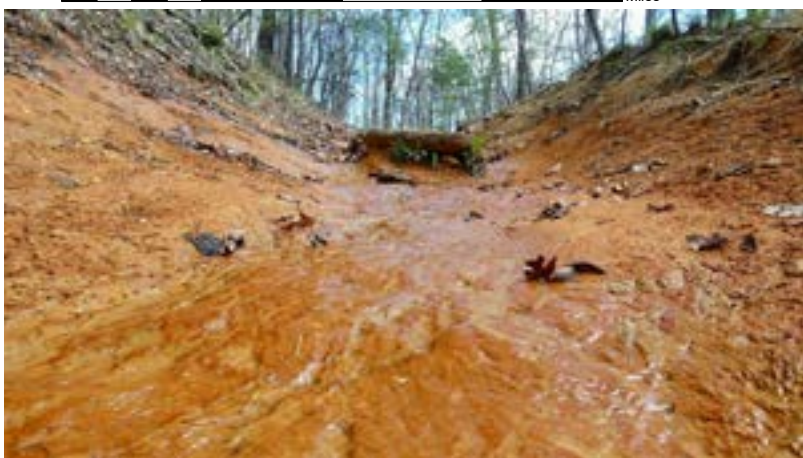
Site conditions include rocky terrain, incompatible soils, and steep slopes
