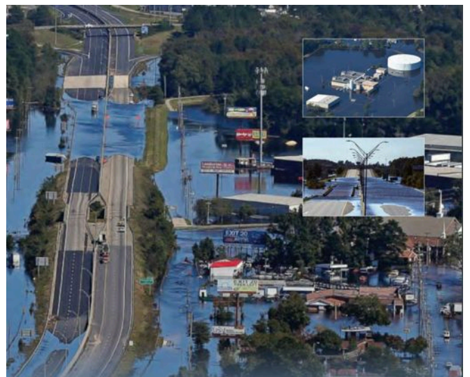
2018 flooding in Lumberton after Hurricane Florence
