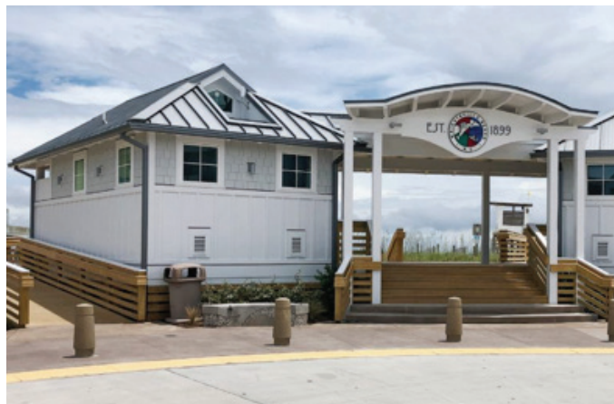
Salisbury Street Restrooms and Access, Wrightsville Beach
