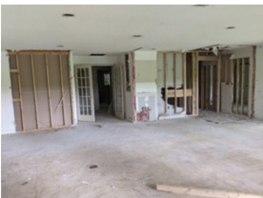
Ranger Headquarters at Lake Julia
