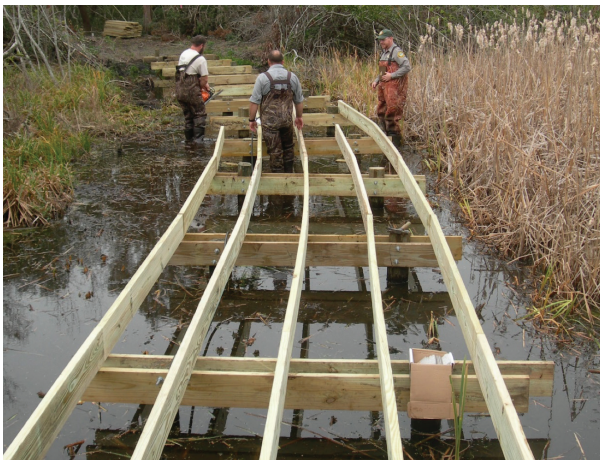
Building the connector trail at Fort Macon State Park
