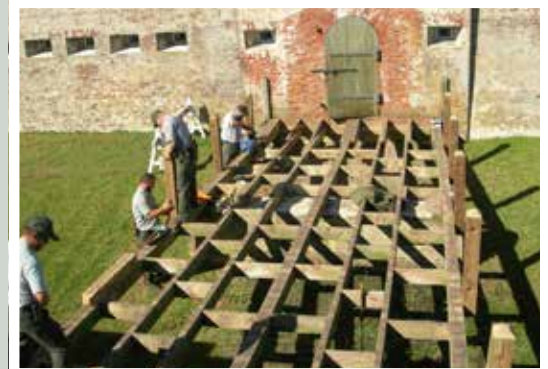
Rebuilding a bridge at Fort Macon State Park
