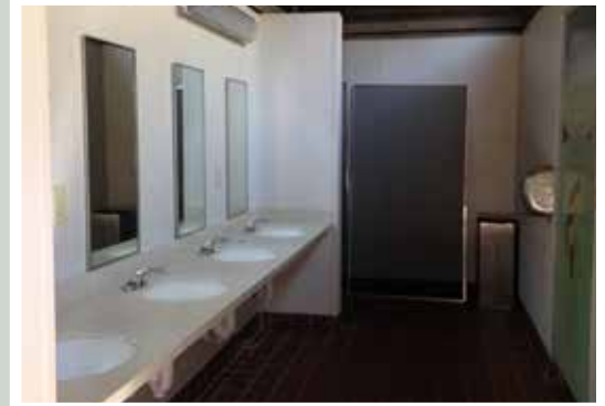
Renovated bathhouse at Poplar Point Campground at Jordan Lake State Recreation Area
