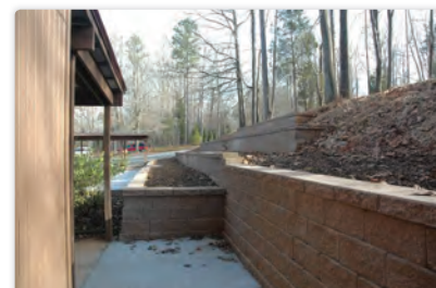
New Retaining Wall
