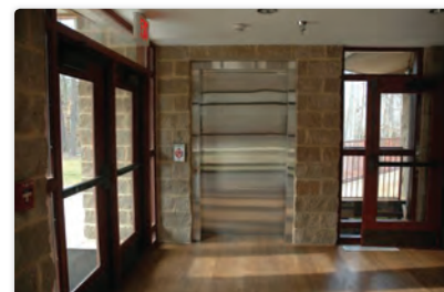
Youth Conference Building Elevator
