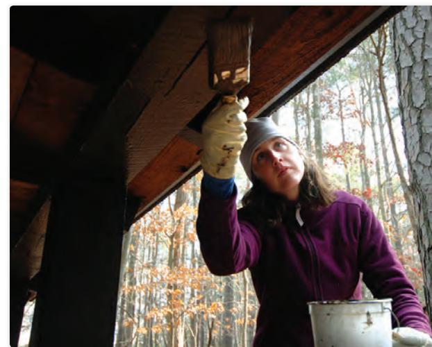
A volunteer helps refurbish facilities at William B. Umstead State Park.
