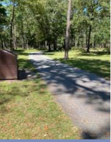
Multi use trail needs to a 1" asphalt overlay in order to be accessible compliant
