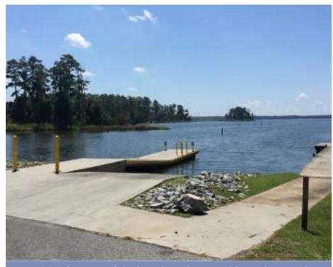
The footings of the boat launch at Dinah's Landing needs a structural assessment performed due to excessive use, current and age.
