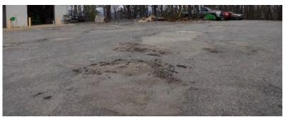
Existing Maintenance area needs grading, re-pavement and paint striping
